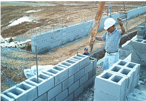
Grout Placement in a CMU wall
